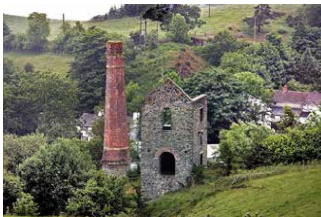
Watson's Shaft engine house at Tankerville Mine. Photo from Shropshire Mines Trust
